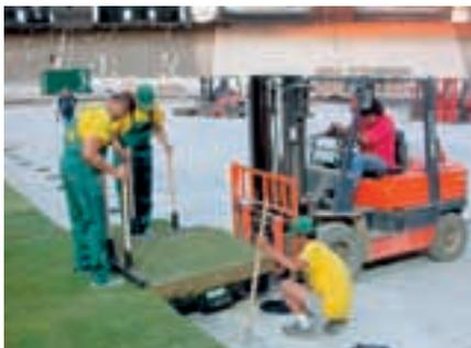
Photo 17: Placement of the locking pad secures the tight contact in-between adjacent modules.
