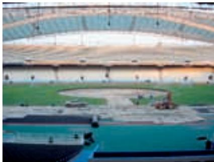
**Photo 26:** Partial removal of the modules from the center of the pitch in order to construct the Paralympic “Tree”
