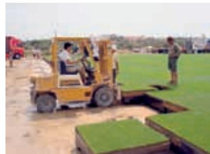
Photo 11: Removal of a module from the established pitch in Spata in order to be transported to the Olympic Stadium.
