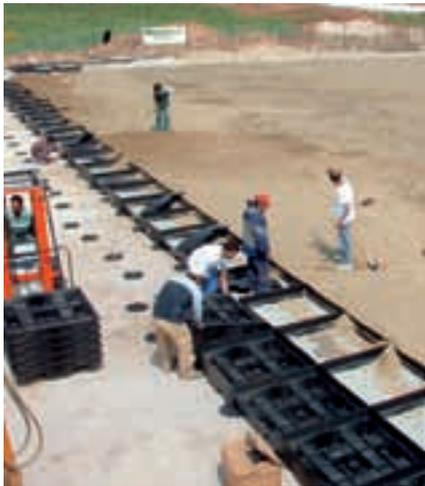
Photo 5: Establishment of modules and filling with the drainage layer and soil substrate.
