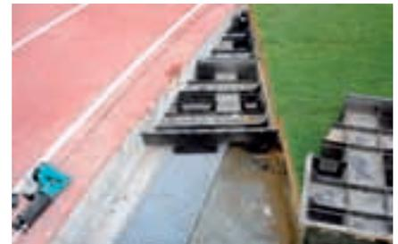
Photo 21: Filling of the curved side of the pitch with the cut modules.
