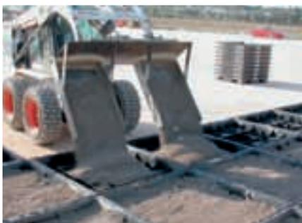
Photo 7: Filling of the modules with the drainage layer.
