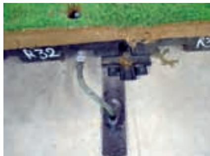
Photo 18: Use of quick couplers for the installation of the sprinklers.
