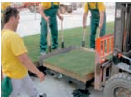
Photo 16: Placement of the module to its final position with the use of metal guides.
