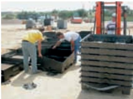
Photo 6: Placement of the sleeve around every other module.
