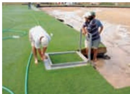
Photo 10: Cutting of the sod and the rootzone is necessary before the movement of the modules.
