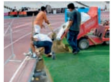
Photo 23: Filling of the cut modules with the appropriate drainage layer and soil substrate.
