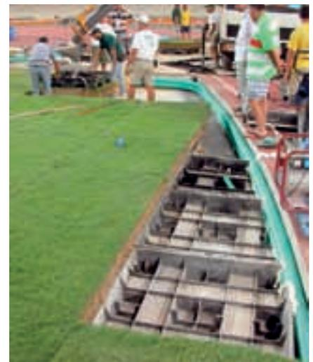
Photo 22: Placement of the cut module in the curved side of the pitch.
